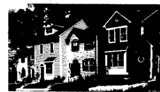
NO RELATIONSHIP BETWEEN FRONT DOOR AND STREET HOOD/SIDE OF MATERIALS. FACADES ARE STAGGERED AND INCONGRUOUS. PARKING LOT IN FRONT OF BUILDING OPEN TO THE STREET.
