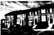
FACADES DO NOT MAINTAIN A CONSISTENT STREET EDGE. PARKING IS INADEQUATE. FRONT DOORS ARE NOT RELATED TO STREET.
